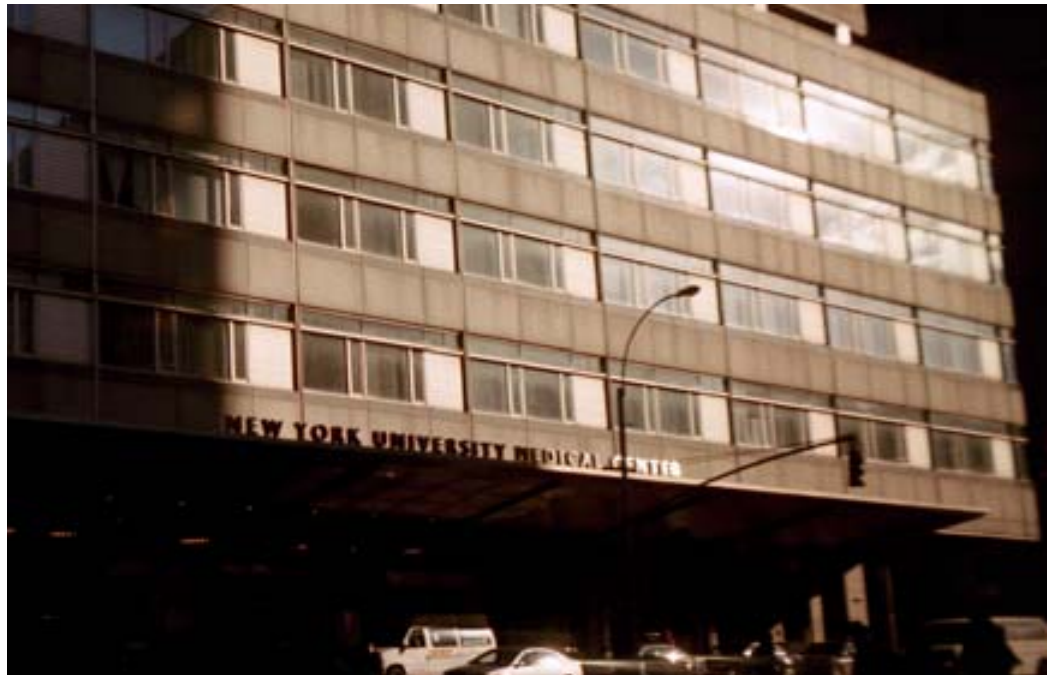
MAIN ENTRANCE OF NYU MEDICAL CENTER
